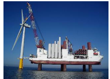
Construction of a turbine off the coast of England.
